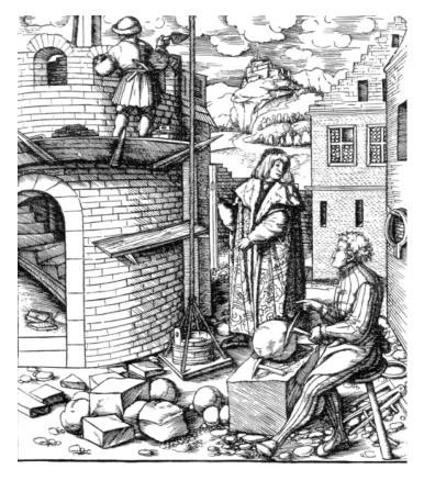
Picture from 1515 showing a "plumb board" or "plumb level". (See also last page)
